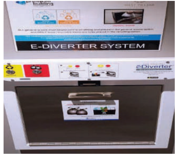
Garbage chutes in the refuse room at West Village, Sydney
